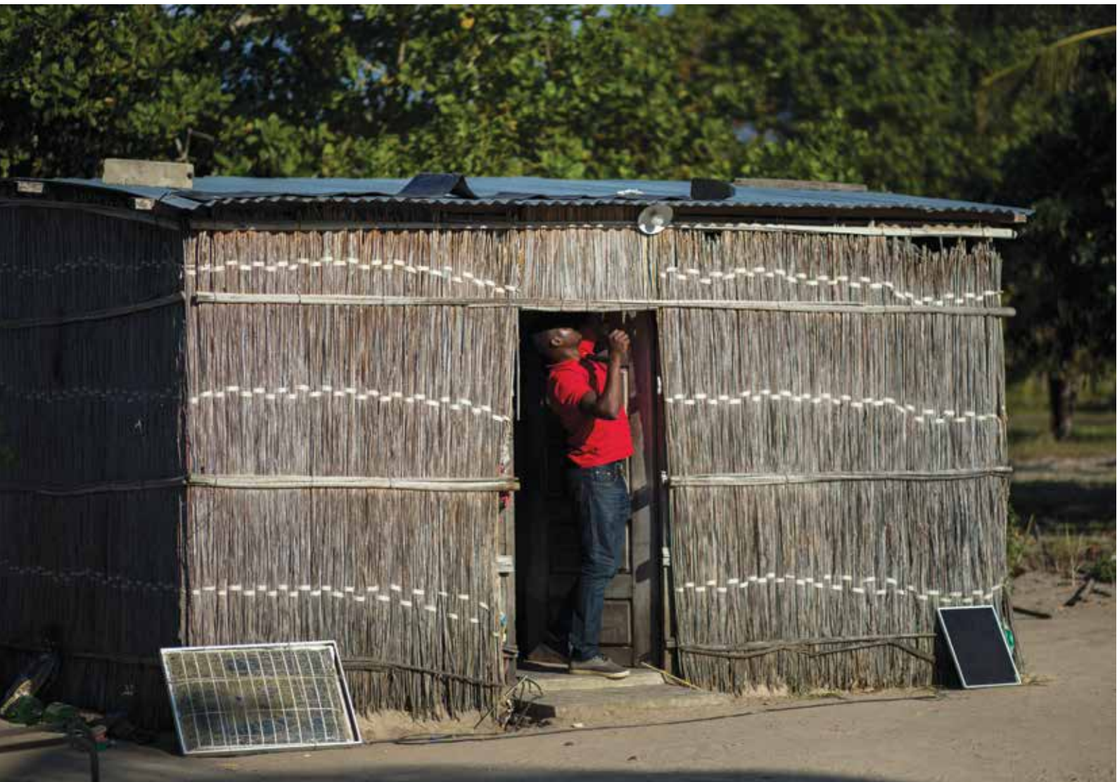
Solar company employee installing a panel (Stefan Freeman, Mozambique, 2018)
