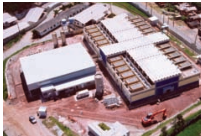
© Unibanco | Usina Bandeirantes thermoelectric plant in São Paulo, Brazil (A view from above), the largest of its kind in the world, delivers substantial amount of carbon credits (see story, p. 52).
