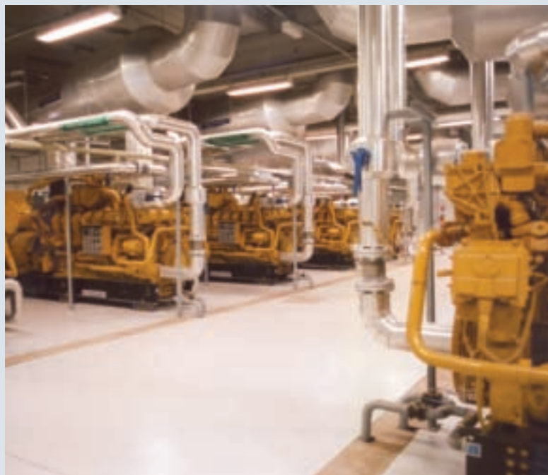
© Unibanco | Usina Bandeirantes thermoelectric plant in São Paulo, Brazil (production facilities) produces clean energy from landfill gas and delivers a substantial amount of carbon credits. The plant is the largest of its kind in the world and was financed by Unibanco.
