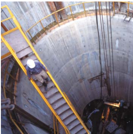
Construction site, Thailand
