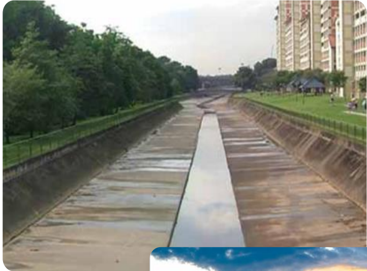
Original concrete- lined canal
