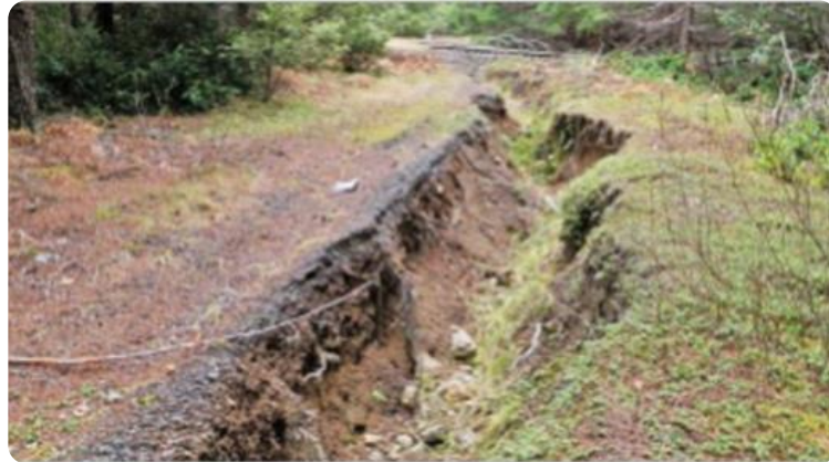
Removal of culverts on an unused road
