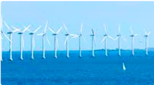
Wind turbines installed with use of ECONcrete 67
