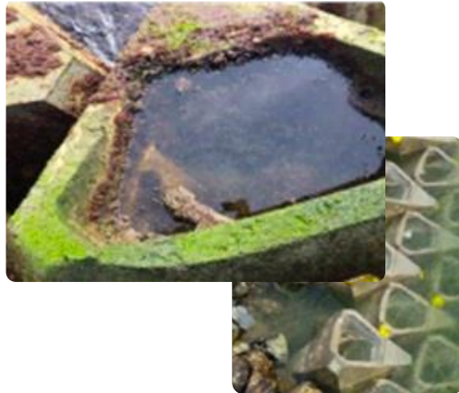
Pilot study of ECONcrete Coastallock armor units in the San Diego port 88
