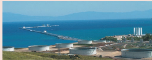
Overview of the terminal with tank farm and jetty.
