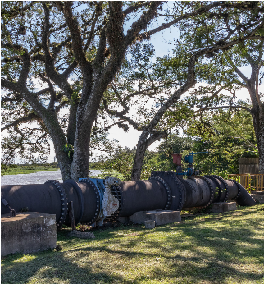
Water catchment station, Brazil Photo: 2022 Marcelo Scandaroli/Illuminati Filmes/IFC
